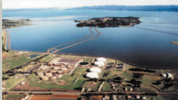
► The oxidation ponds will be opened to the sea and 13 kilometres of coastal edge restored.
