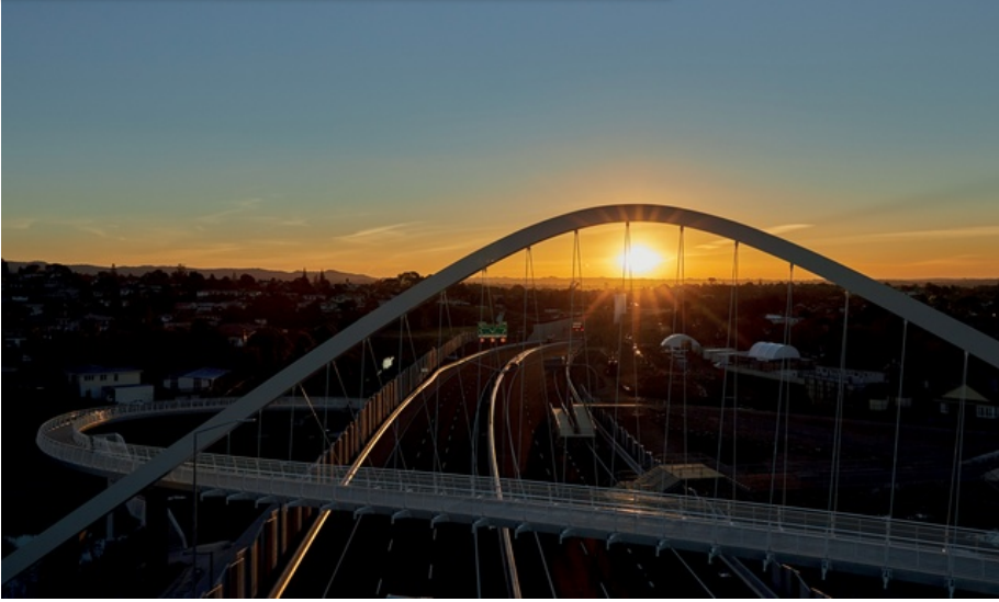
Te Whitinga pedestrian bridge spans the motorway, referencing Auckland's maunga with three pure arcs. Image: Ariel Camera
