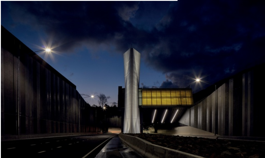
Night-time view of the southern ventilation building. Image: Sam Hartnett
