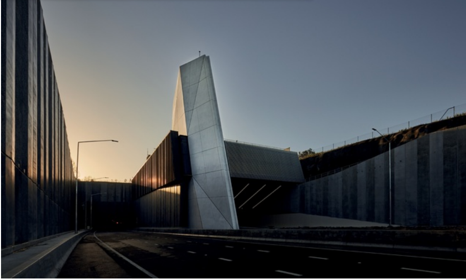
The western elevation showing the southern ventilation building. Image: Sam Hartnett
