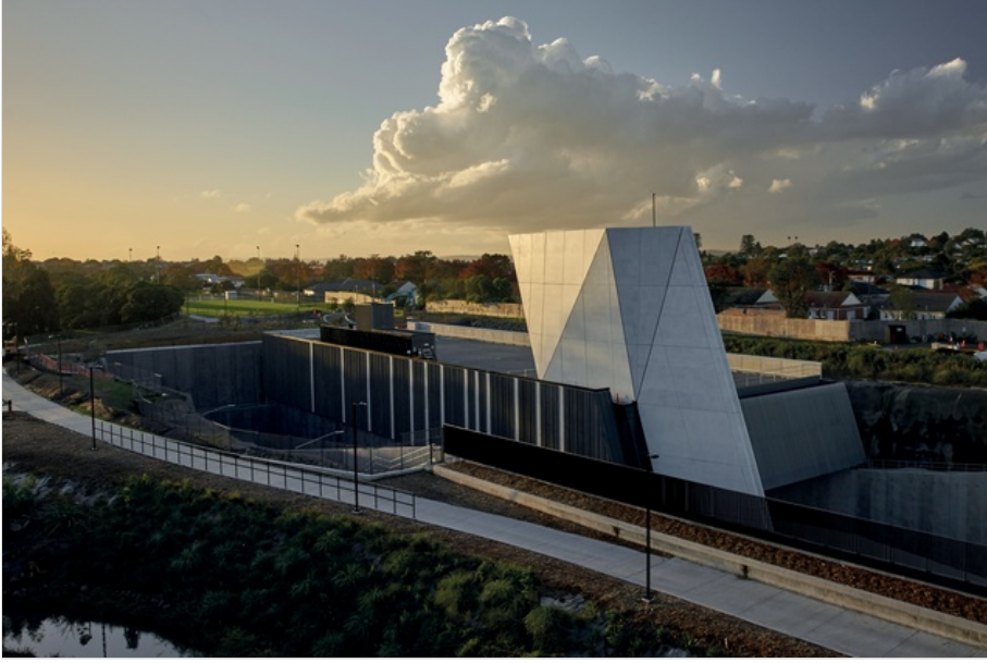
The motorway approach into the Waterview Connection's 2.4km-long twin tunnels. Image: Sam Hartnett
