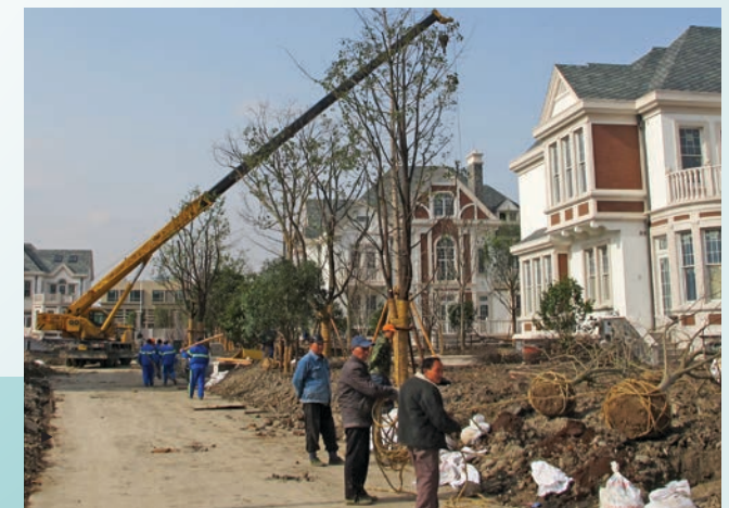
Specimen trees are lifted into place at Dong Jiao Villas at the start of the planting season, March 2013.
