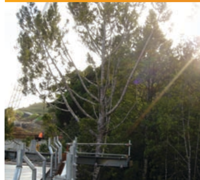
▲ A 150-year-old kauri stands tall beside the Otenurua viaduct, intact thanks to the construction crew calculating beam placement with precision.
