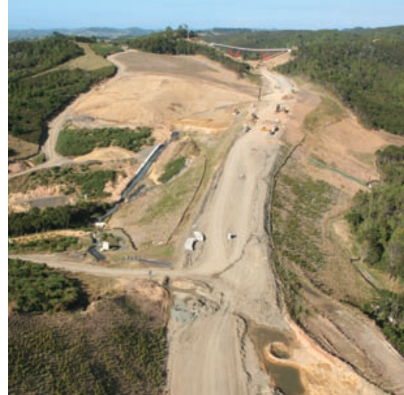
▲ Steepened batters, such as the newly planted foreground slope, have preserved 4ha of forest edge along the motorway route.
