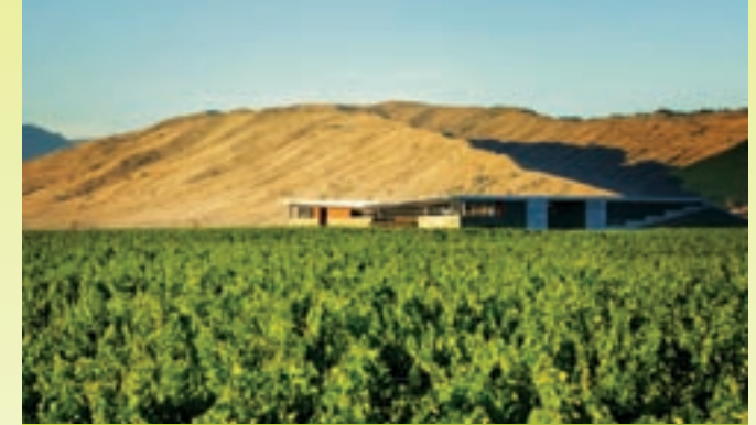
▲ Influenced by the landscape: Ara's 'Dart' operations building was designed by Warren and Mahoney in collaboration with the master planning team, with Boffa Miskell also designing the 'oasis' garden and immediate landscape context.
