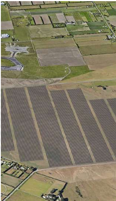
▶ Kōwhai Park Solar Farm
