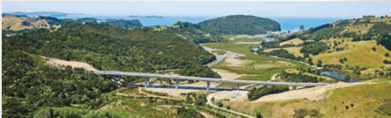
▲ Traversing sensitive areas: the Waiwera estuary (centre) and the Johnstone's Hill twin tunnels (left) where the portals were extended to allow revegetation instead of massive retaining walls.
