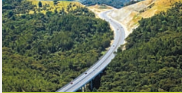
▲ Native forest remains intact below the Otanerua eco-viaduct. Instead of horizontal benching, cut batters merge into the existing landform (top right).
