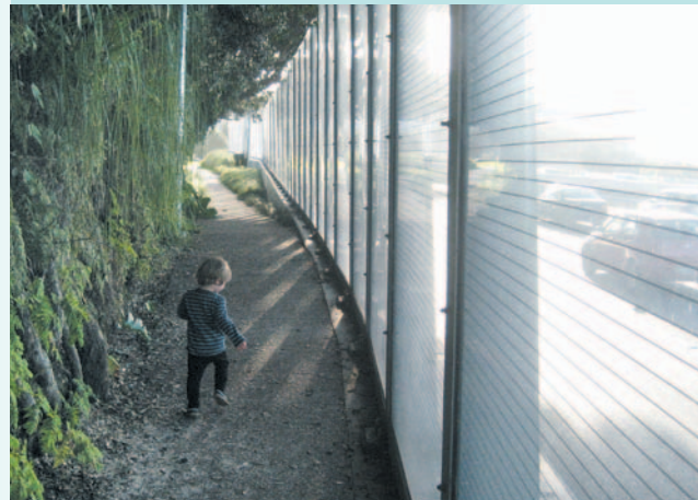
▼ The transparent wall buffers traffic noise whilst allowing motorists to see the pohutukawa-clad cliffs (left) that once overhung the original shoreline.
