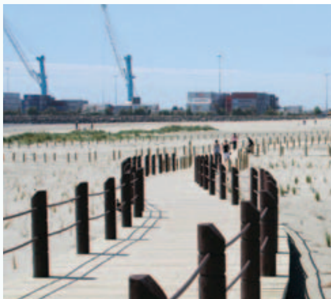
▲ The Caroline Bay boardwalk provides easy access and protects native dune enhancement plantings (Timaru port in the background).
