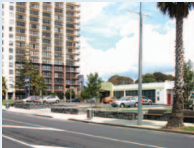
▲ Improvements to Sharkey Street will act as a catalyst for future investment in the area.
